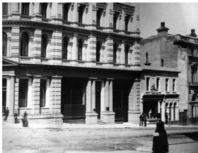
Above left: Wilkinson's tiny shop next to the huge AMP building on the corner of Dowling & Princes Streets, late 19th century.
