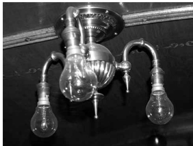
Top: Roslyn number 1 tram, new and ready for action – Otago Witness 31 October 1900. Middle: The tram carcass in the Museum's NZR Garage awaiting final restoration, 2006. Bottom: An example of one of the missing electroliers – photograph supplied by Dave Carr of the Heritage Tramways Trust.
