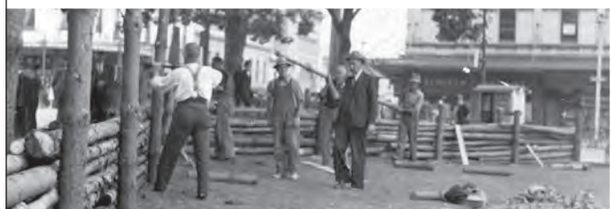
Palisaded trenches under construction in the Octagon, 15 December 1941 - courtesy Allied Press
