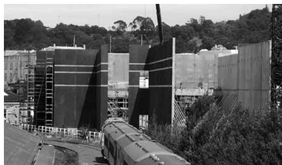
The new collection store begins to take shape.
