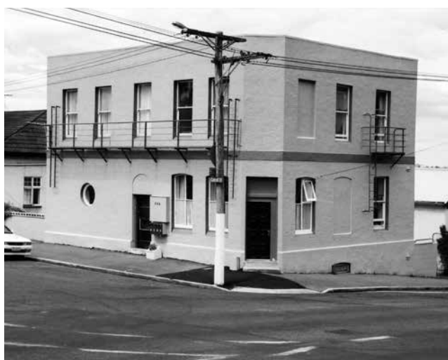
The Apollo Hotel building today, situated on the corner of Carroll and Maitland Streets
