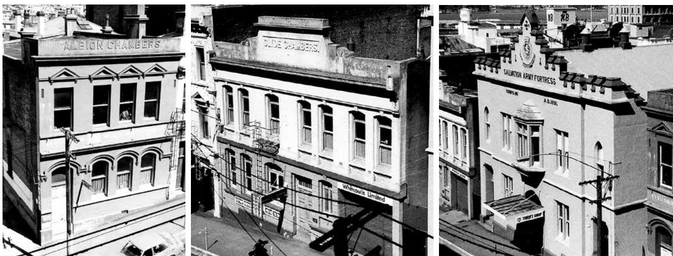
Left to right: Albion Chambers, Clyde Chambers and the Salvation Army Fortress circa 1980 – New Zealand Historic Places Trust Otago Branch Archives [27 August 2007].
