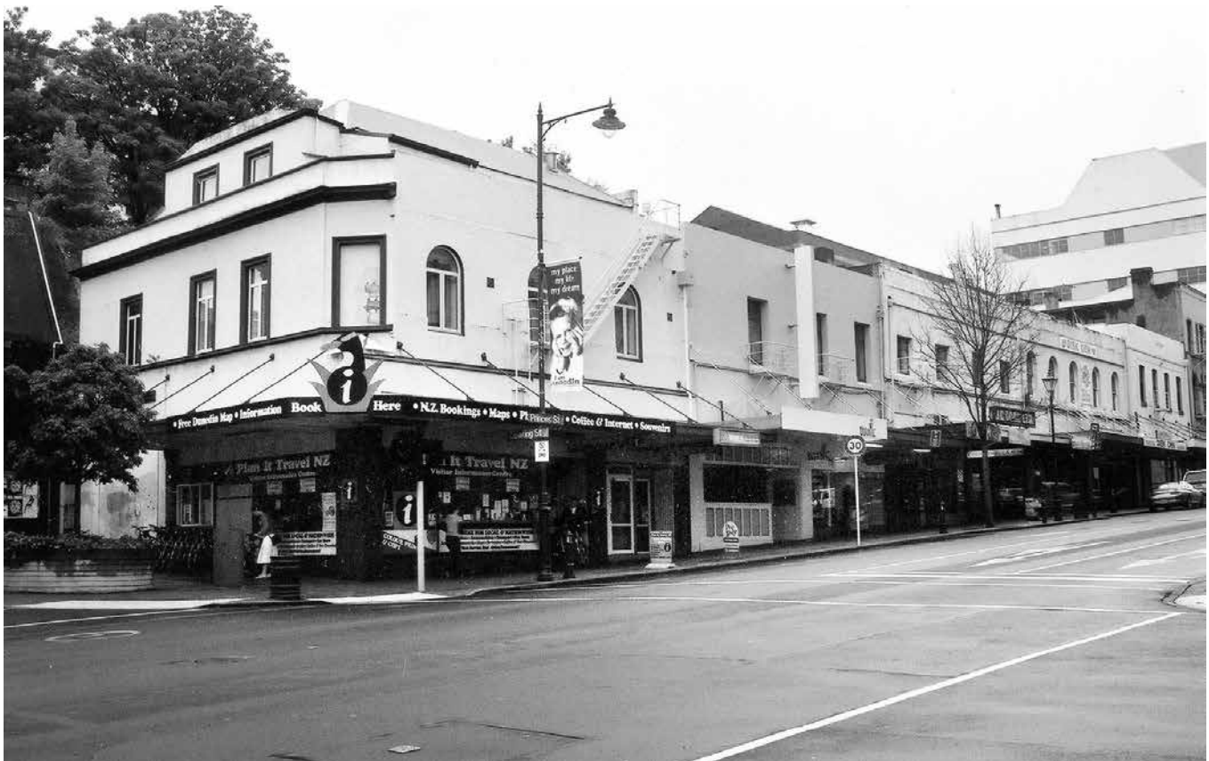
Farley's Buildings today – Many of the windows have lost their original arched form and most of the decorative brickwork has been covered.
